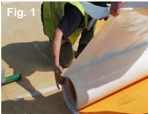
Fig. 1 - Peel away approximately 12 inches of release paper from the Stickymat adhesive layer
