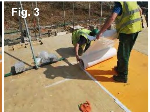
Fig. 3 - Working in pairs, roll out the mat progressively whilst peeling away the release paper. For large areas, use a dry roller to smooth out.
