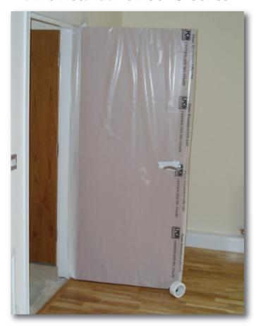
Manufactured from fully accredited LPS 1207 polythene, Flame Retardant Door Sleeves allow all types of doors, single, double, standard and fire doors to remain in operation whilst preventing cosmetic damage.
