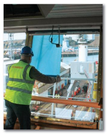
Ockwells Flame Retardant Hard Surface Protection Film has been developed to protect doors in areas under construction and refurbishment. This protection is manufactured from flame retardant polythene film with a special low tack adhesive back that is designed to protect hard surfaces on a temporary basis without leaving a residue.
