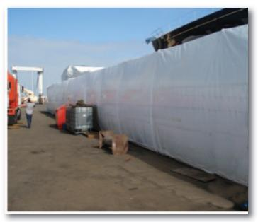
Manufactured from reinforced low-density opaque flame retardant polythene sheeting.
