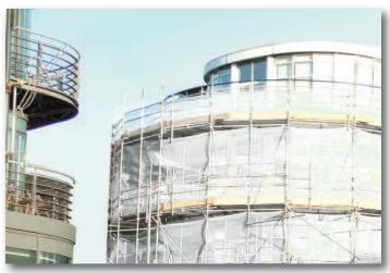
Knitted fabric with button hole eyelets for easy installation, designed to improve site safety by reducing the risk of small objects or tools falling outside the work area.
