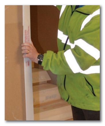
Flame Retardant Edgeguards and Stair protectors are made from TwinShield which is certified to LPS 1207.
